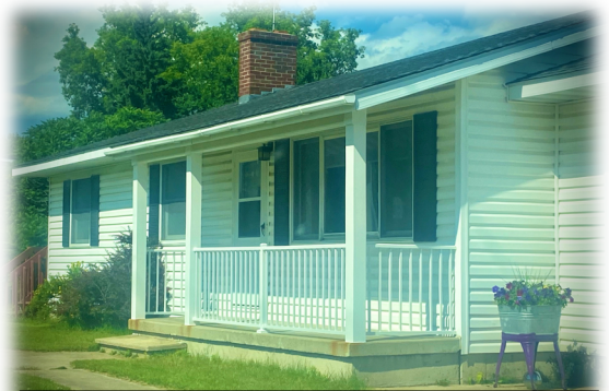
Be sure to check-out the newly installed porch/railings at the Parsonage. No more worrying if the awning will fall down during heavy winds with supports as strong as these!
